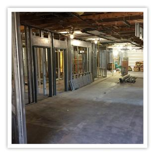
framed and plumbed with those walls nearly complete; structural demo is complete; steel supports for roofing have been installed; new vestibule area foundation has been laid and rough framing is underway; HVAC new fan coil units and ductwork have been installed in the education wing; electrical rough-in continues; AVL rough wiring is complete, including stage and sound booth. Wi-fi cabling is being installed by our volunteers.
